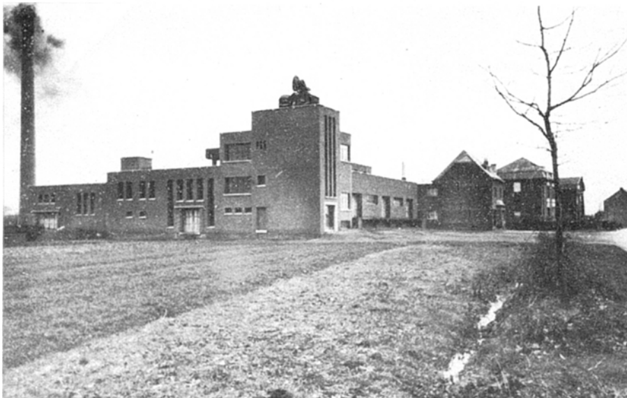
Complete trailer assembly mounted on roof of dairy building at ZONHOVEN.
